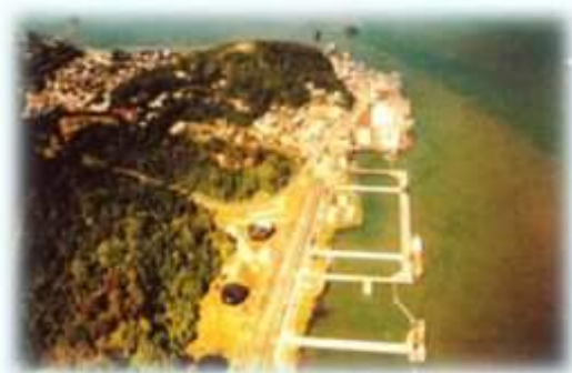
Balikpapan Port, East Kalimantan (1988-1992) Construction Supervision.
