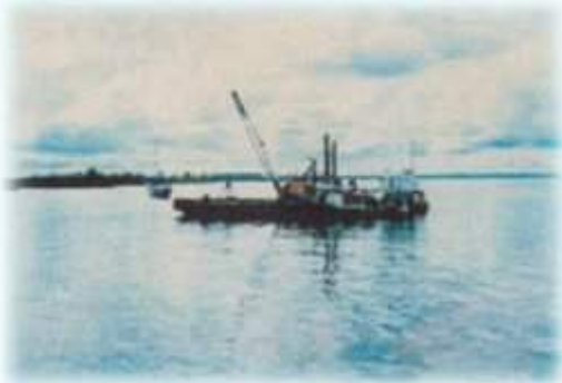
Banjarmasin Port, South Kalimantan (1988-1989) Supervision of Dredging Work
