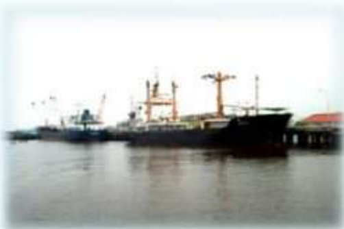
Dumai Port - Phase III, Riau (2001-2007) Master Plan, Detailed Design and Construction Supervision
