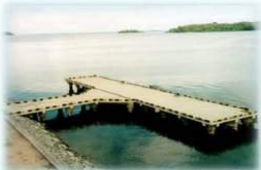
Seget Port, Sorong, Papua (1995-1998) Detailed Design and Construction Supervision
