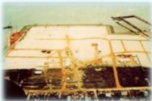
Dumai Port - Phase I, Riau (1989-1990) Construction Supervision of Reclamation.
