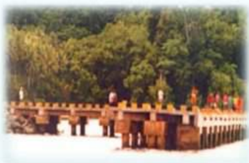
Numfor Port, Papua (1994-1997) Detailed Design and Construction Supervision.
