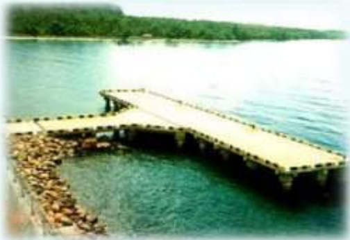
Ransiki Port, Manokwari, Papua (1995-1998) Detailed Design and Construction Supervision
