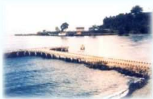
Maumbawa Port, East Nusa Tenggara (1995-1998) Detailed Design and Construction Supervision
