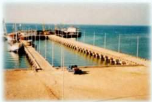
Reo Port, East Nusa Tenggara (1994-1997) Detailed Design and Construction Supervision
